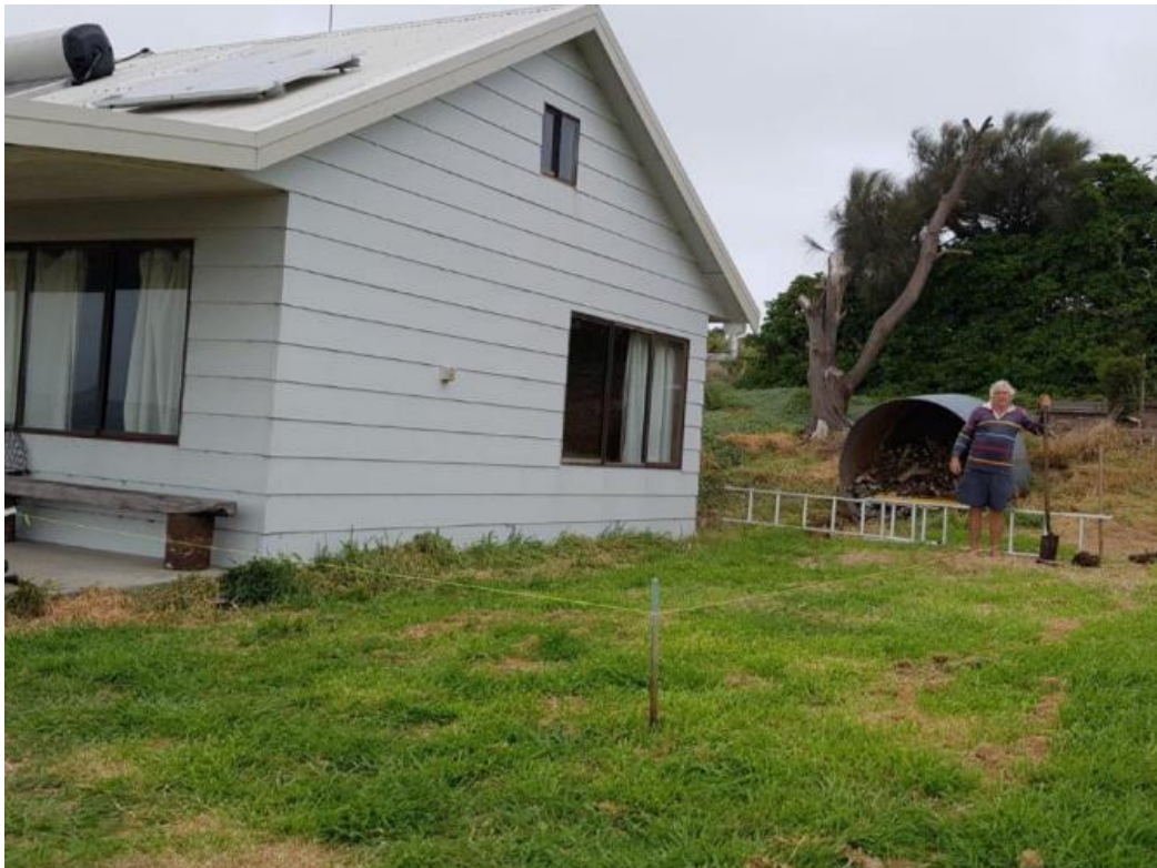
Photo 4 Photograph showing extent of the proposed additional building footprint
