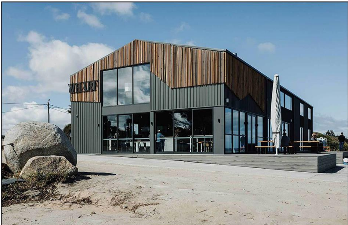
Photo 3: As constructed Flinders Wharf building northwestern perspective, decking and windows on western side overlooking the Whitemark Wharf.
