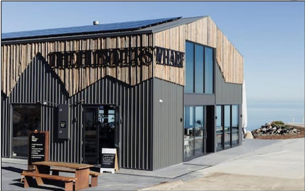
Photo 2: As constructed Flinders Wharf building northeastern perspective, main entry point on eastern side.
