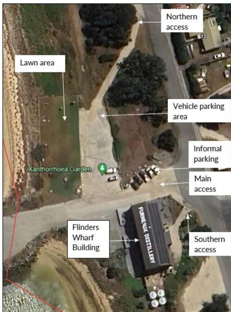
Figure 9. Aerial photograph showing the existing building, vehicle parking area, lawned area and information parking and access 16 Esplanade, Whitemark, March 2024
