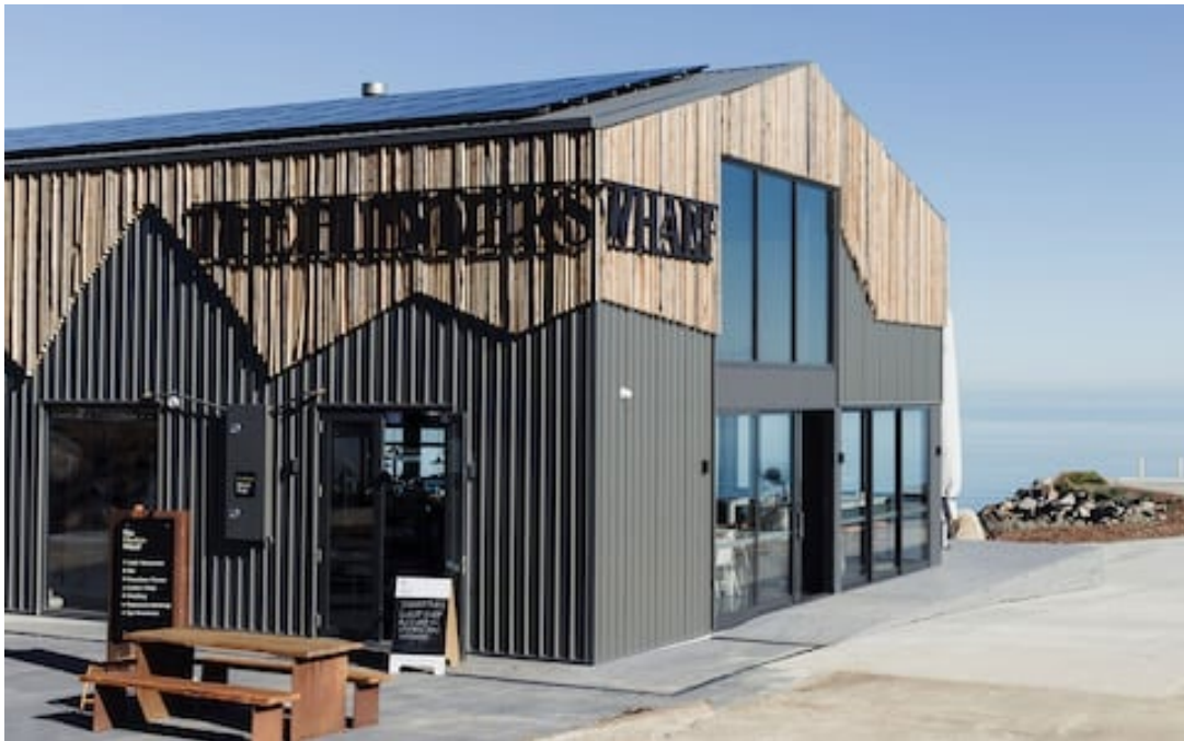
Figure 2: Existing building view of eastern and northern facade
