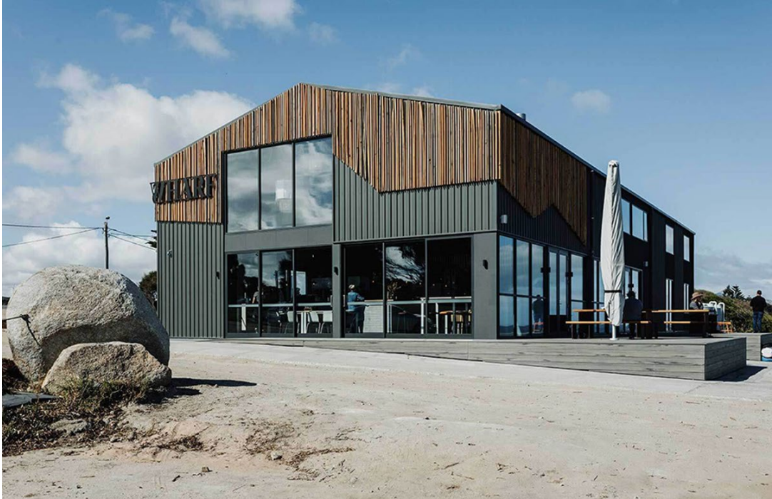
Figure 3: View of the northern and western façade
