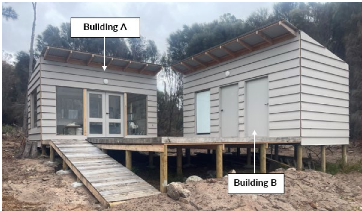
Figure 5.4 – Building A B deck cluster – image taken in February 2025 by Council staff.
